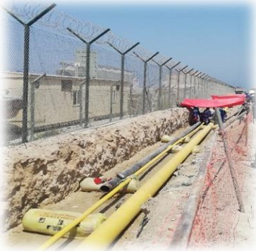
Underground pipeline works
